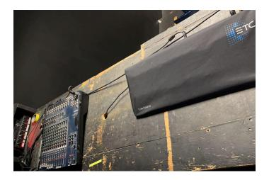
The on-off switch for the light board is on the back of the board, to the right of the monitor. To power up and down the audio system: turn on the mixer 1st, then the processor, then the power amplifier last. The reverse is true to power things down. Turn the power amplifier off 1st, then the processor, then the mixer. Also, the lighting control console should be powered off each day and any
